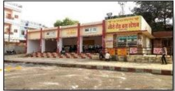
Passenger waiting area & enquiry counter
